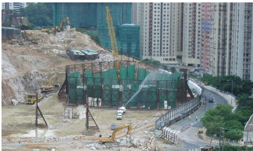
Gambar 2.6. Pemasangan Vertical Screen and Cages
