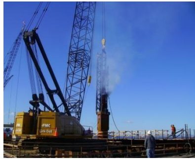
Gambar 2.11 Diesel Hammer
