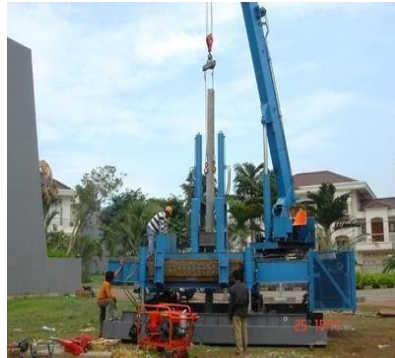
Gambar 2.12 Hydraulic static pile driver
