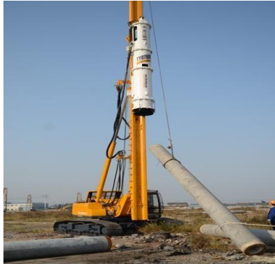
Gambar 2.10 Drop Hammer
