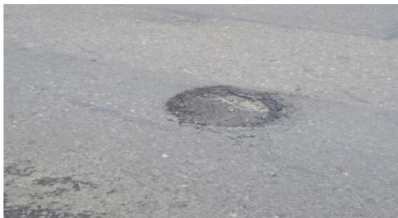
Gambar 2.13 Lubang ( potholes )
