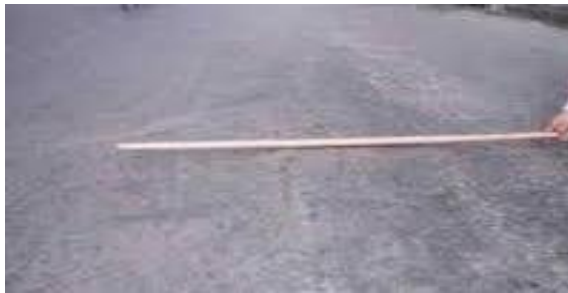
Gambar 2.12 Jembul ( upheaval )
