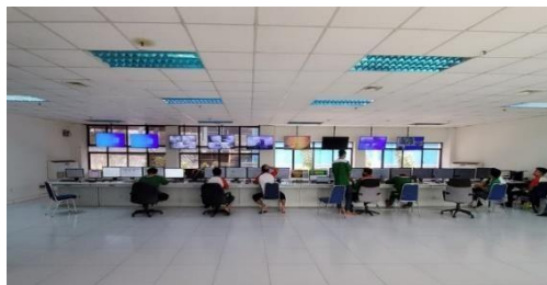
Gambar 2.14 Central Control Room (CCR) Pabrik PT. Semen Baturaja
