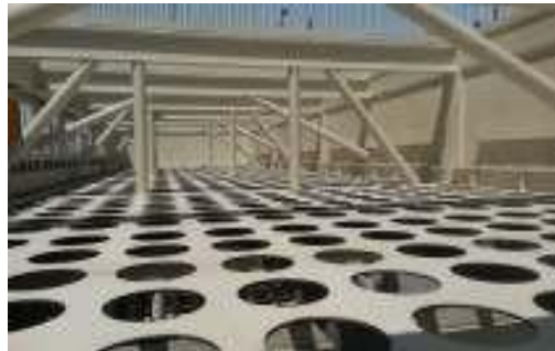
Gambar 2.5 Tubesheet (AAF Instruction – Bag Installation)
