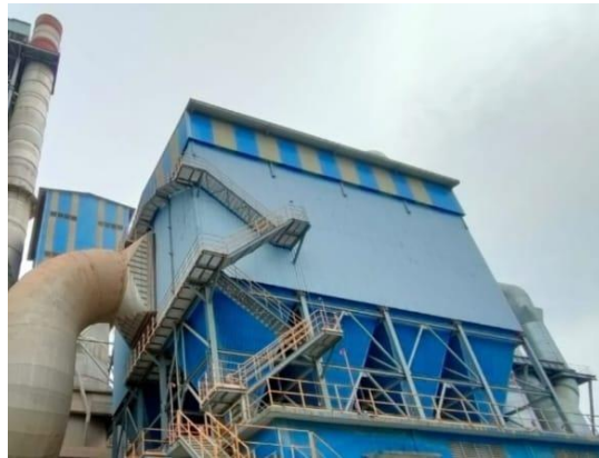
Gambar 2.1 Bag Housing (Widcahyono, 2022)
