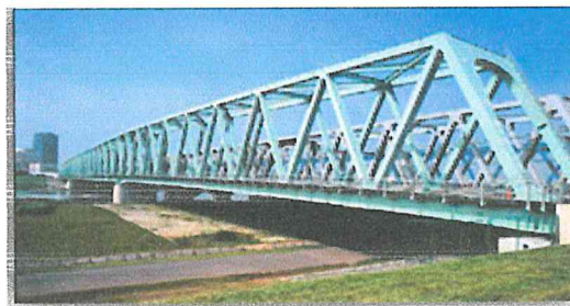
Gambar 2.2 Tipe Warren Truss
