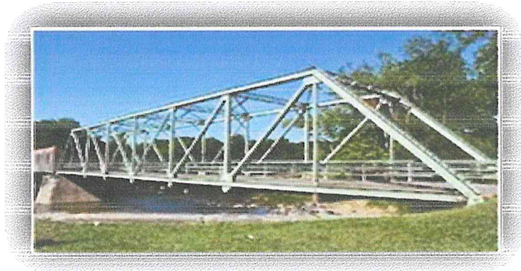
Gambar 2.3 Tipe Pratt Truss
