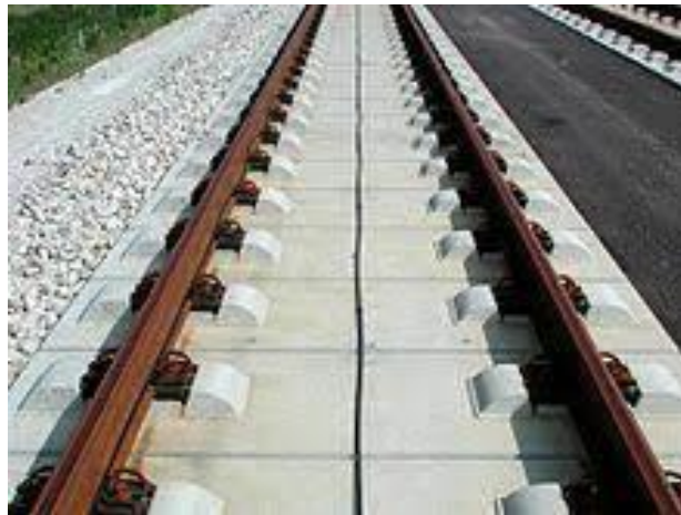
Gambar2. 9 bantalan slab
