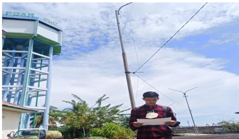
Lokasi Menara Reservoir PDAM OKU
