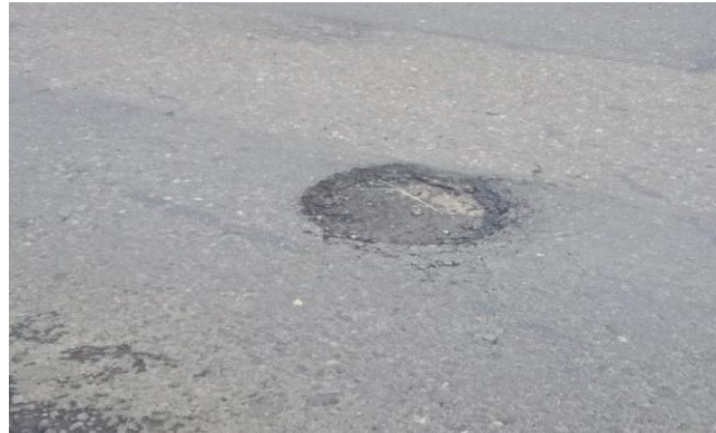
Gambar 2.5.17 Lubang ( potholes )
