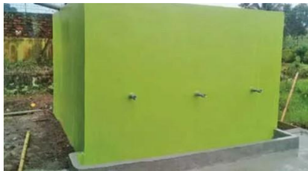
Gambar : 2.12 Reservoir Pasangan Bata
