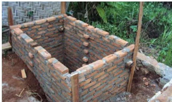
Gambar : 2.12 Reservoir Pasangan Bata
