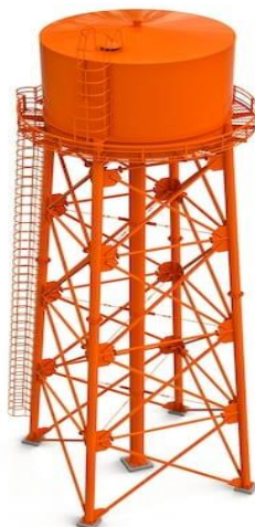
Gambar : 2.9Reservoir menara air (Elevatedreservoir)
