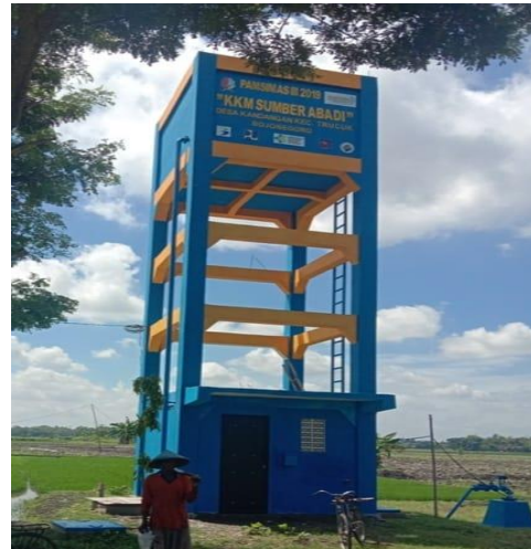
Gambar : 2.9Reservoir menara air (Elevatedreservoir)
